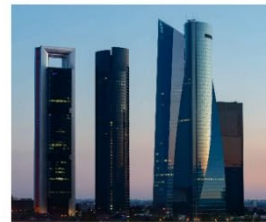
International Building Decarbonization Conference 2024 Madrid, Spain
