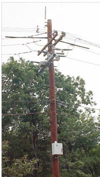
Figure 2-1. ASU Placement on Overhead Line
